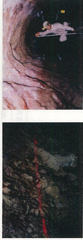
Headrace tunnel without concrete lining
